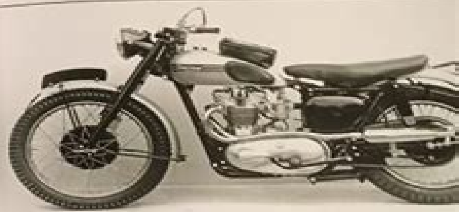
For the 1954 500cc TR3, the factory motor was fixed with right lock front fork.
